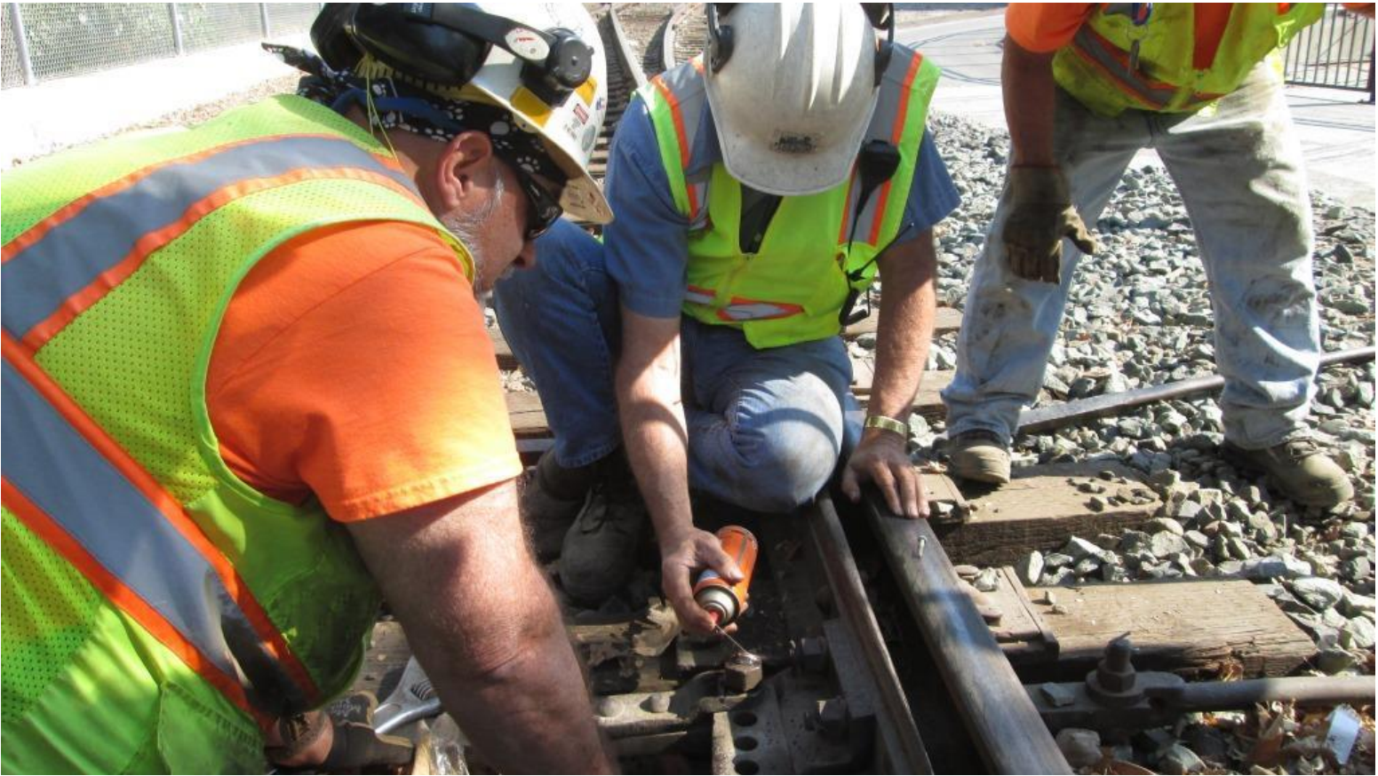
Alan sprays magical Kroil on the bolt connecting the connecting-rod to the transit clip
