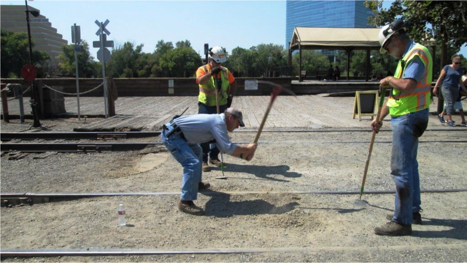
DSLE Jeremy finds the concrete under center-siding that he remembers being there when they laid the track in the 1990s
