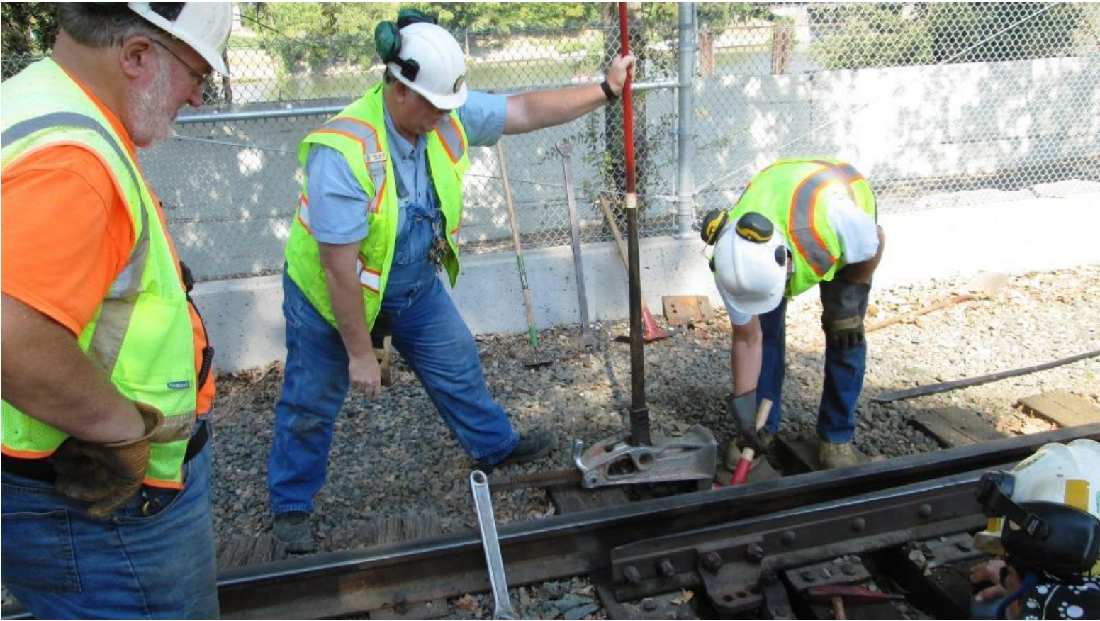
Chris slides a tie with the track-jack as Clem knocks a plate into position
