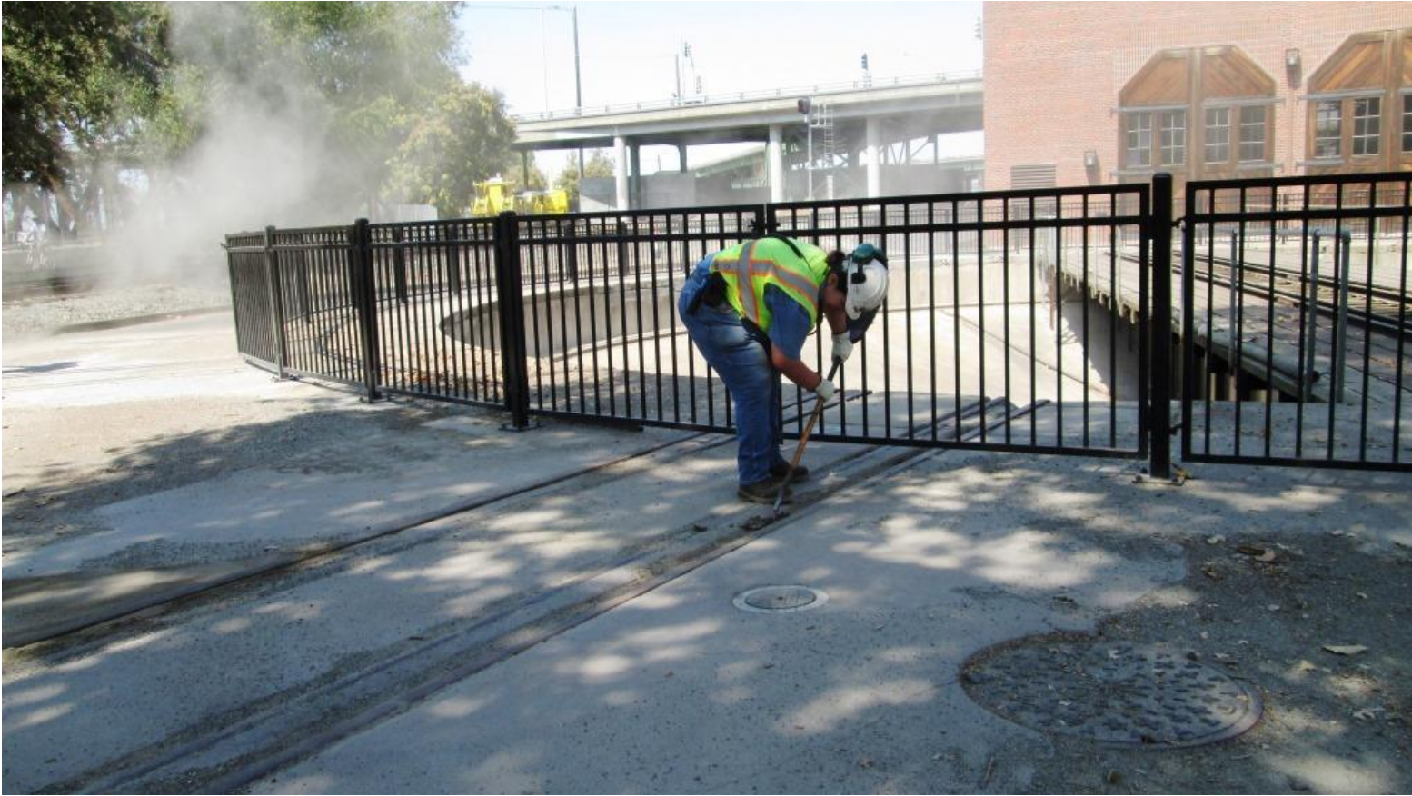
Heather scrapes compacted dirt out of the flange-way of the North Turntable Lead
