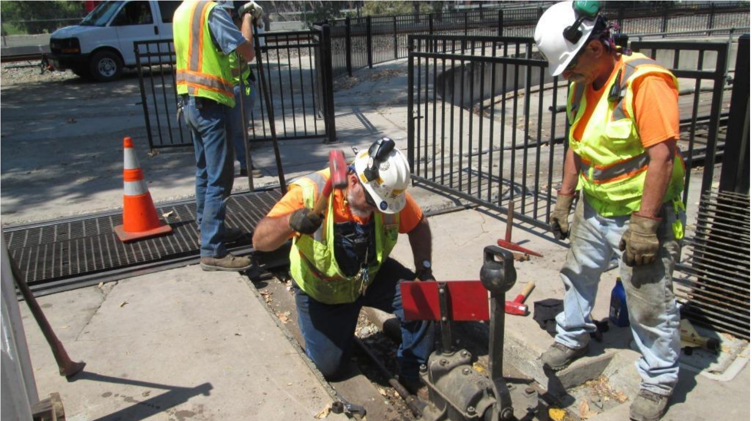
Heather and Matt use lining-bars to hold the points at the measured-mark as Mike F. spikes-down the switch machine
