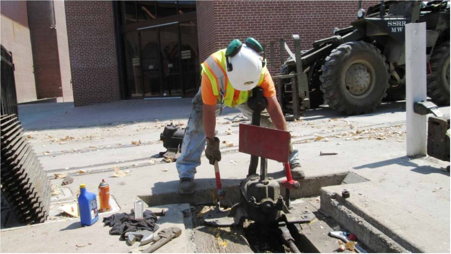
Joe uses his patented double-fisted sledgehammering technique to make minute adjustments to the position of the switch machine
