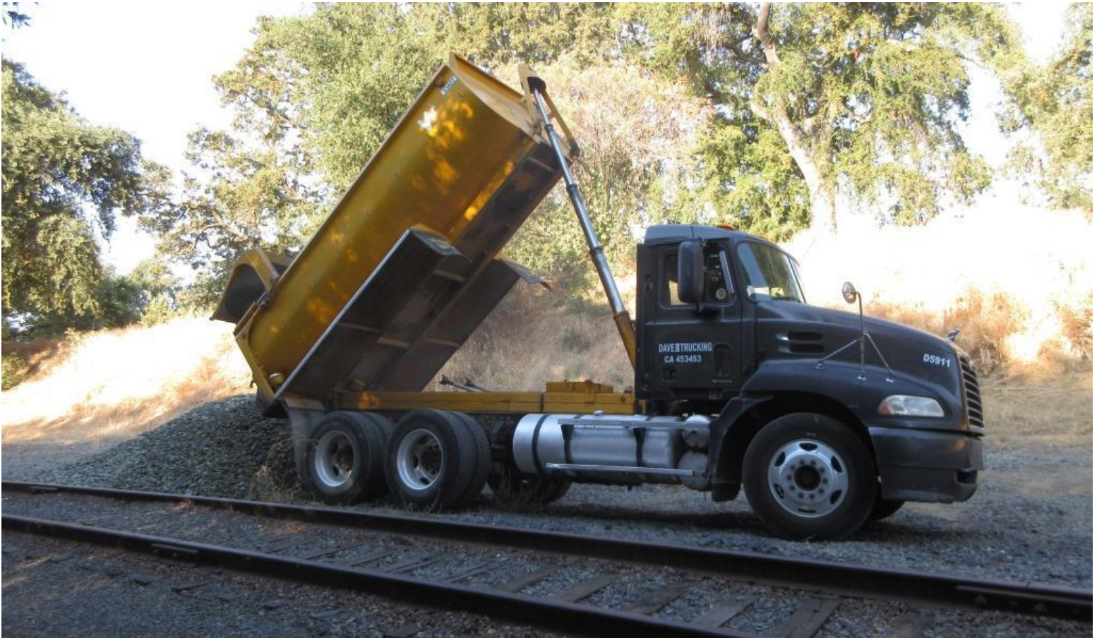
And work throughout the day, Mount Ballast grew!
