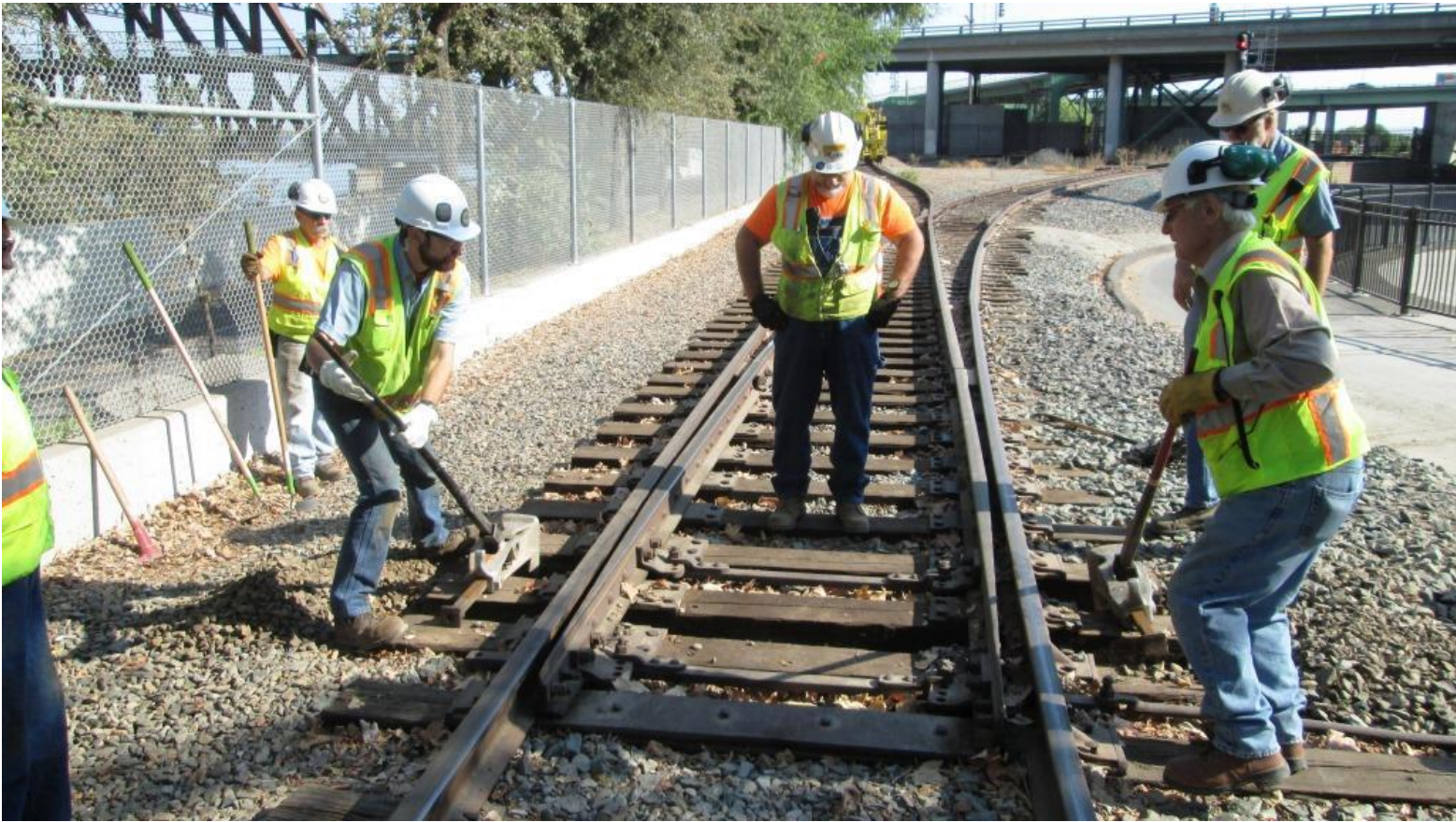
With jacks laid horizontally, Matt and Mike W. start cranking on them to push the offending tie south
