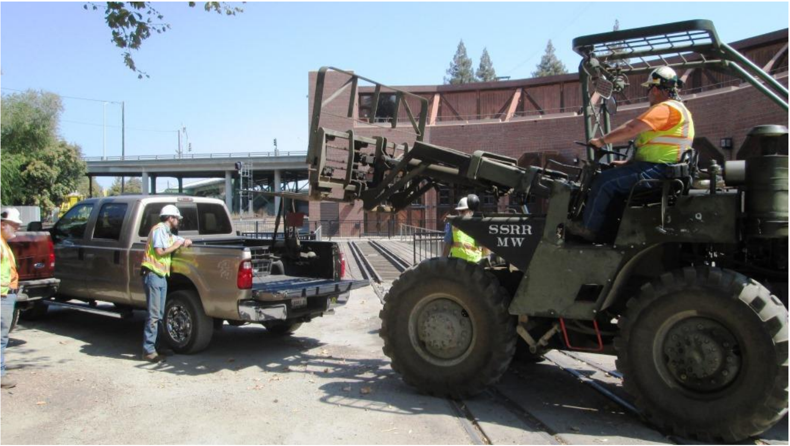
Mike F. on Big Green grabs the replacement switch-machine
