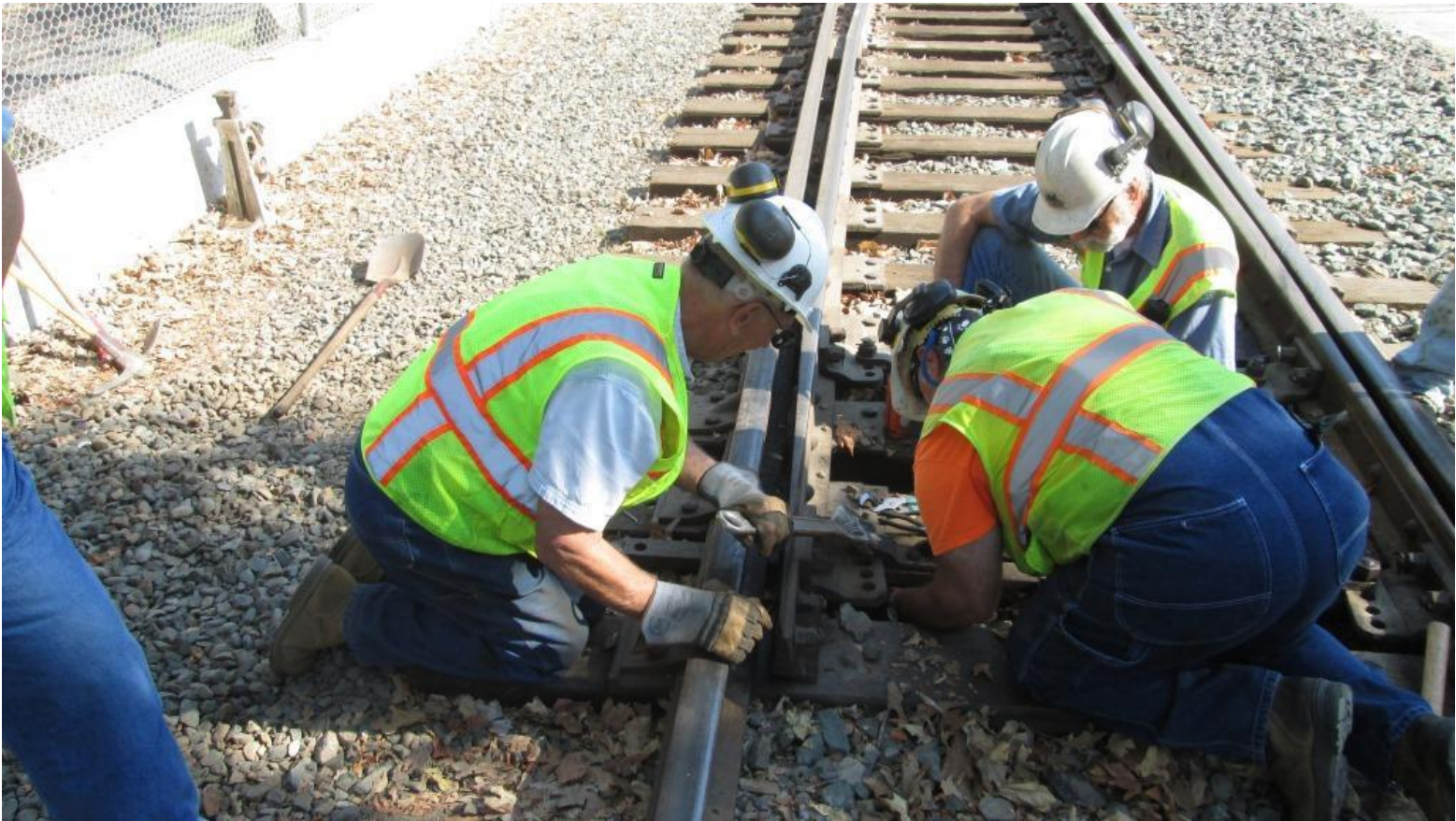
Now to the other side where Clem, Mike F. and Alan make adjustments to the connecting rod at the transit clip
