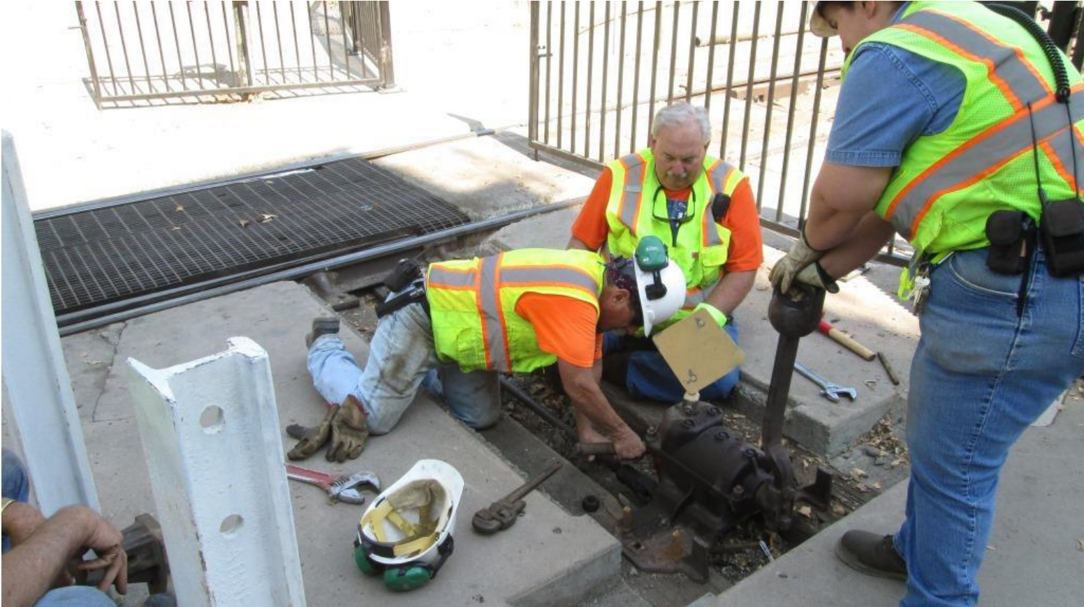
Joe, Harry, and Heather disconnect the switch-rod from the switch machine
