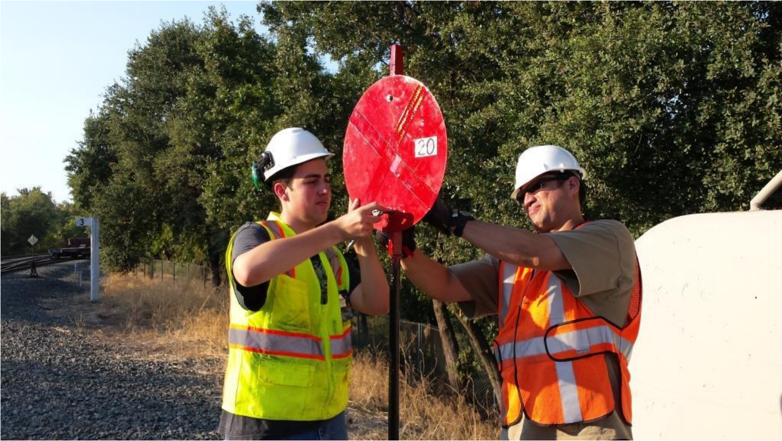
Weston and Jose make repairs to the switch machine at Switch 20
