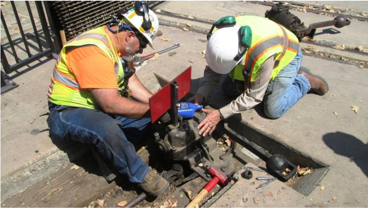
Mike F. adds oil to the switch machine while Mike W. uses his thumb as a dyke against spillage
