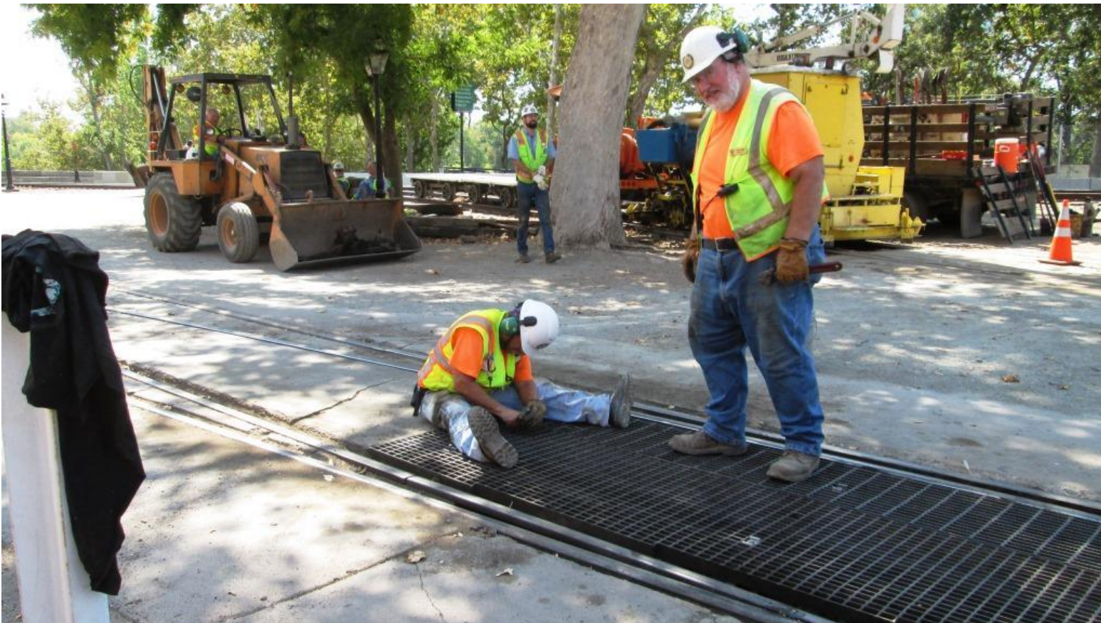
Frank and Joe blots down the grating over the switch
