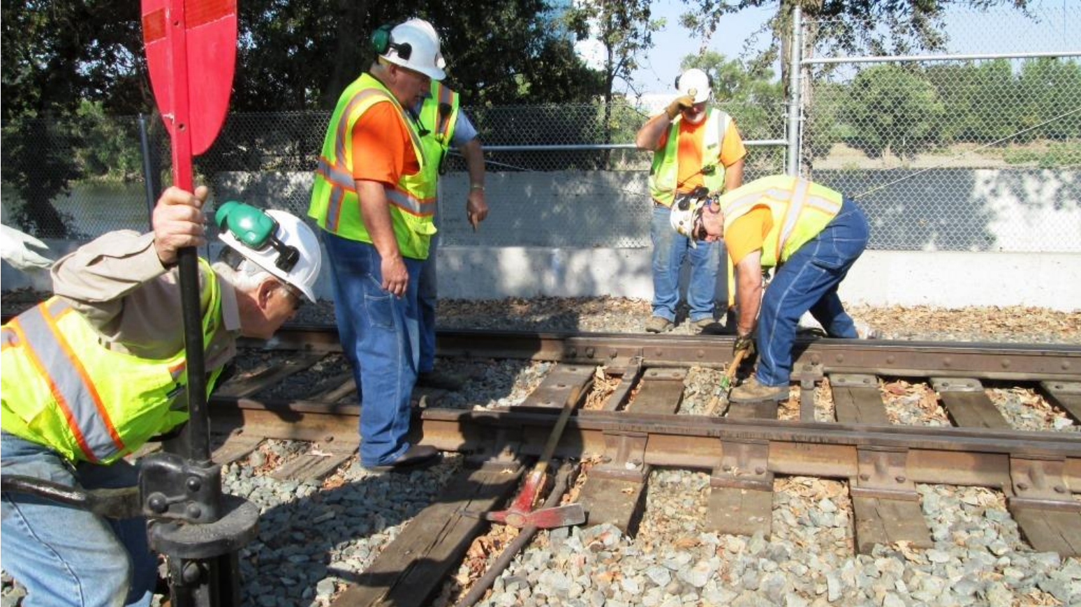
Mike W. floats the switch-points as Mike F. begins digging out the ballast next to the tie to be moved
