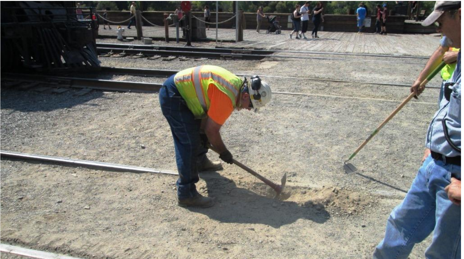
Mike F. surveys under the platform track
