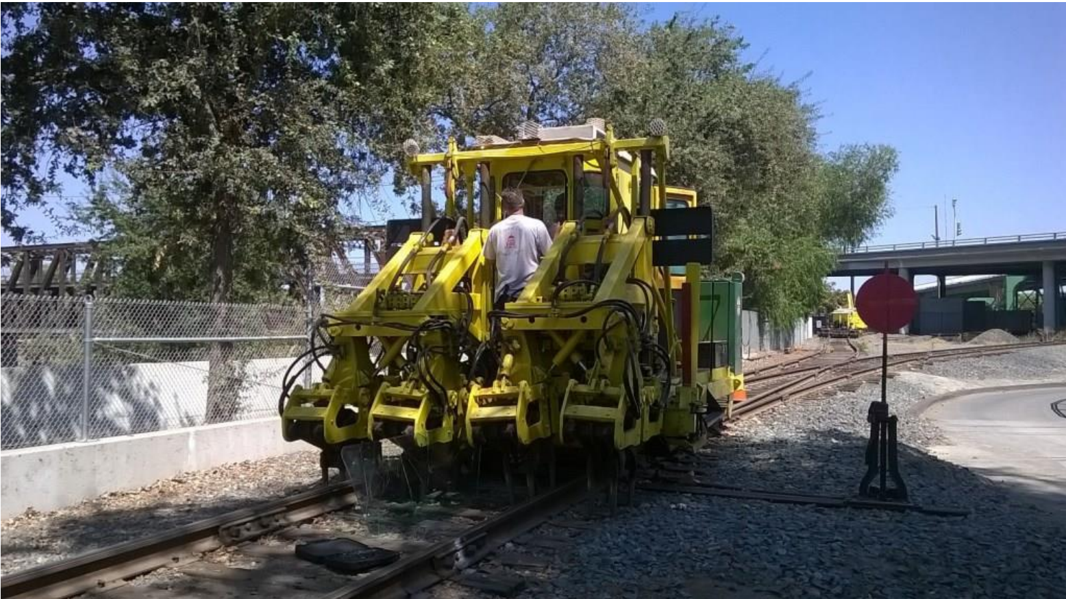
The windshield of the tamper is replaced
