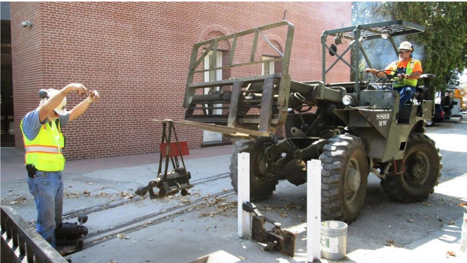
Alan guides Mike F. on Big Green for the placement of the replacement switch-machine
