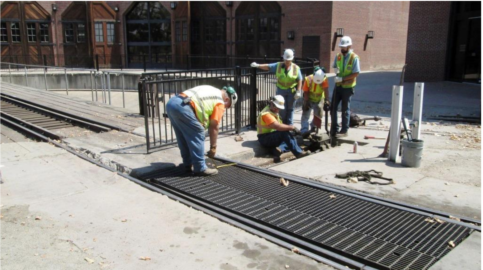
Adjustment of the switch begins with centering the switch-points. Frank measures as Joe manipulates the machine to center the points
