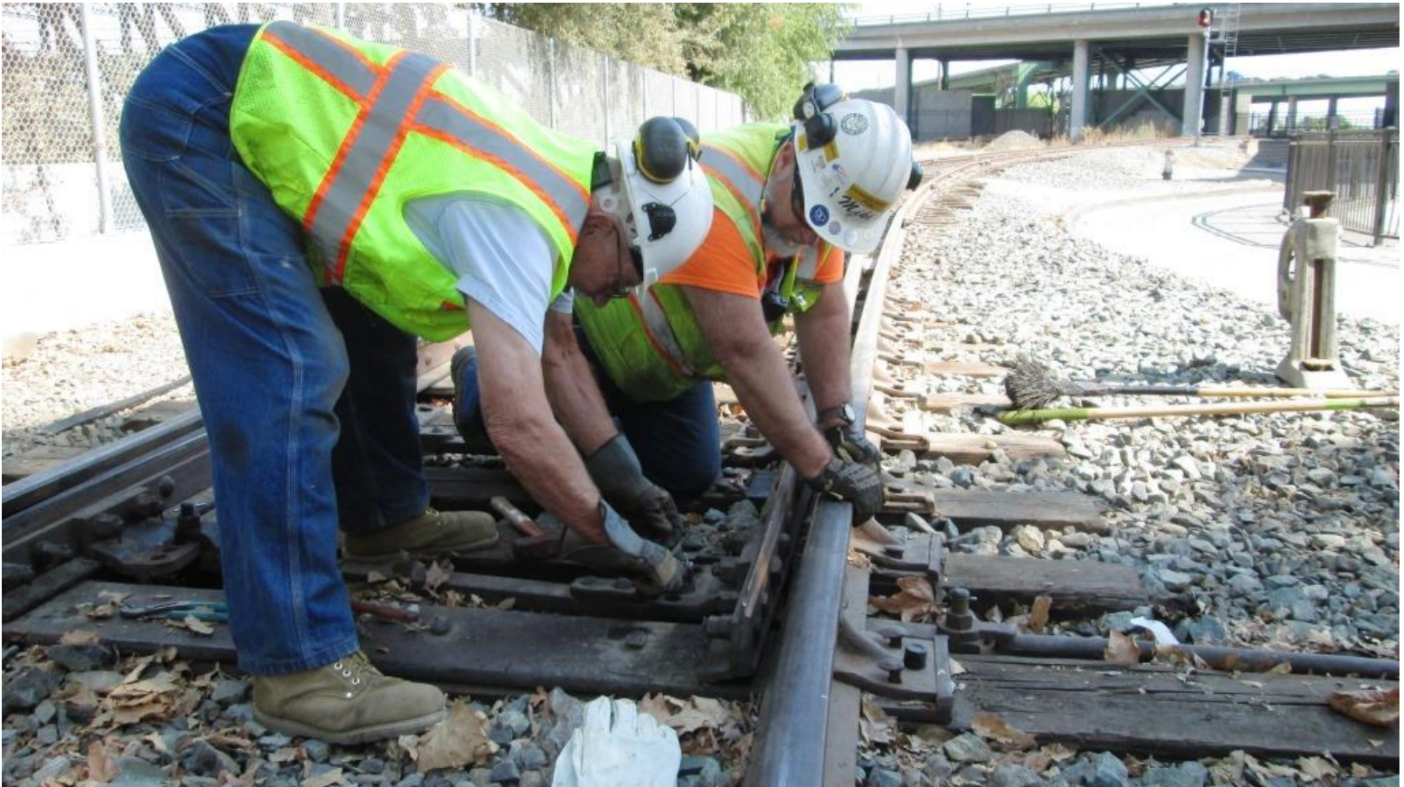
Clem and Mike F. tighten-down the connecting rod in its new position
