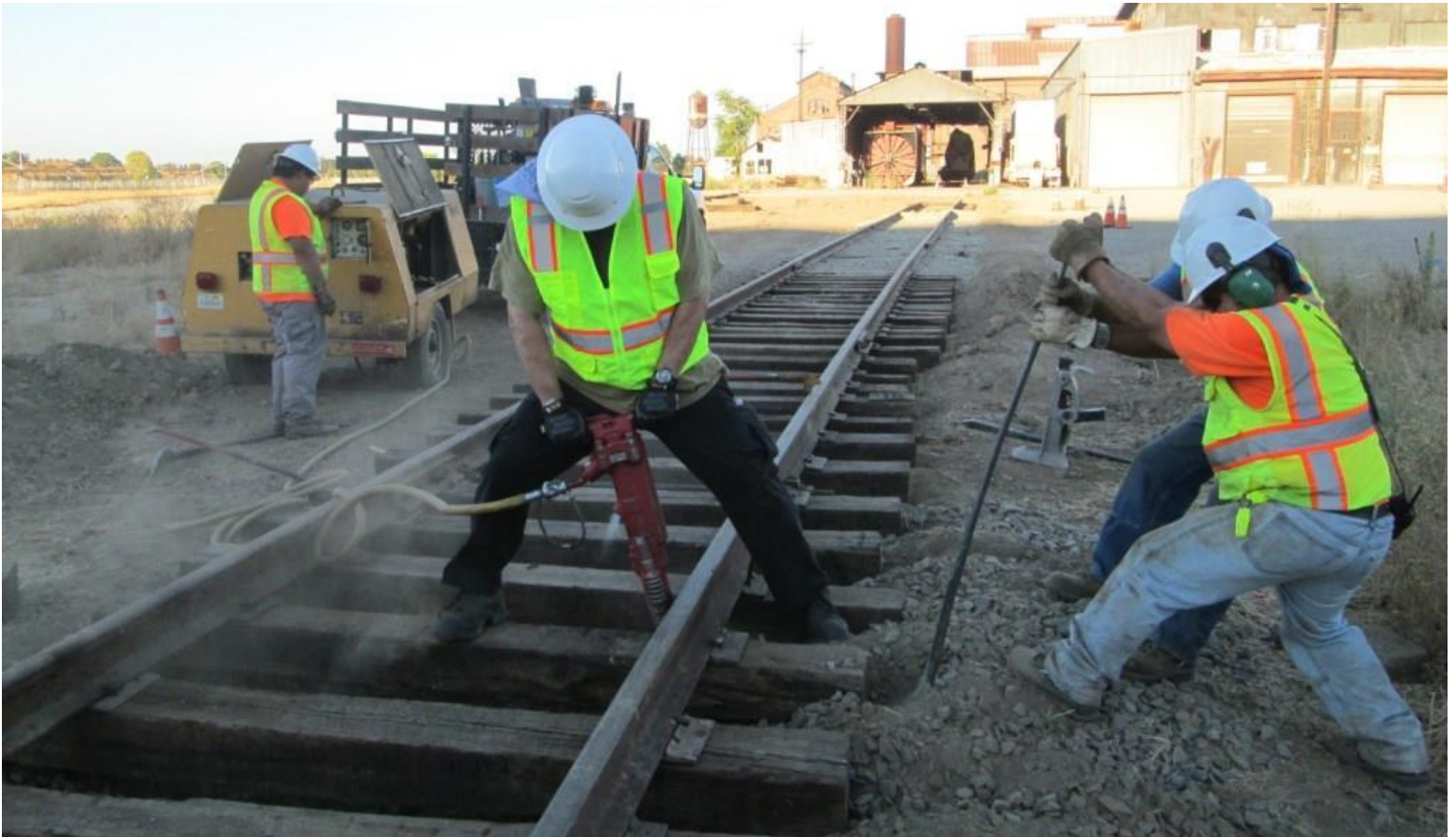
Jose drives spikes as Ed and Joe pull together to nip-up the tie
