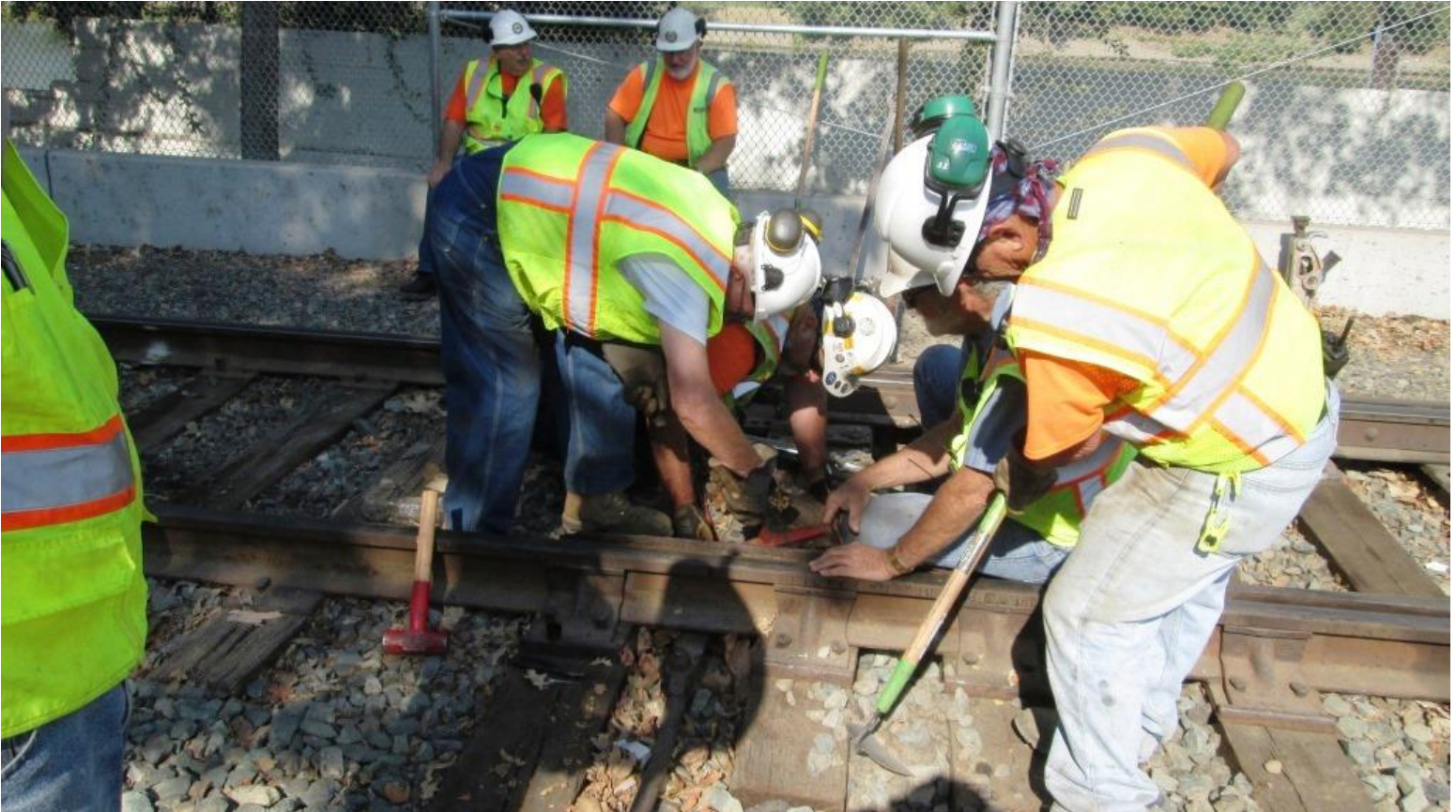
Clem, Mike F., Alan, and Joe work on the adjustment of the switch
