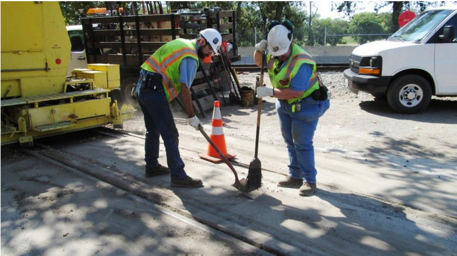
Matt and Heather clean up from their flange-way scraping
