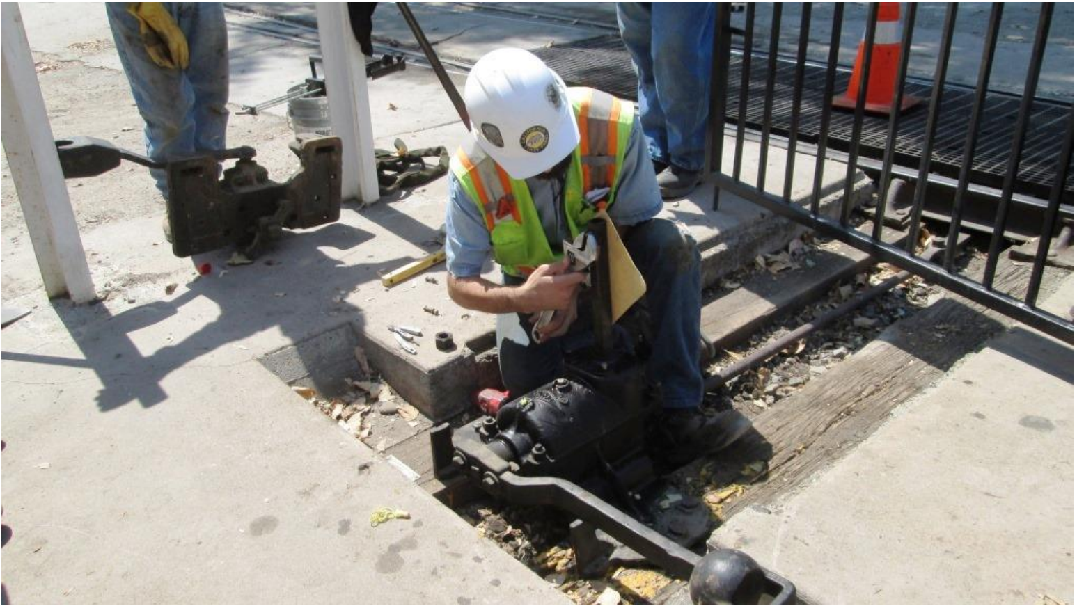
Finishing touches on the switch-machine switch-out: Matt installs the proper target
