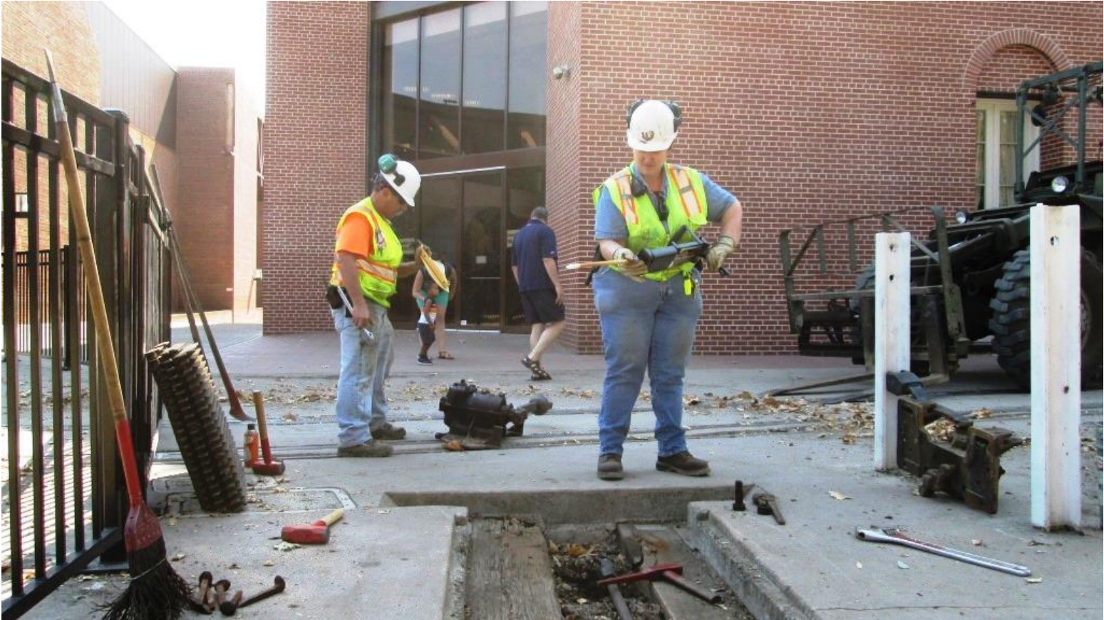
Locked and loaded! Heather prepares to shoot special epoxy-goo into the cracks and crevasses of the cracking and crevassing switch-tie
