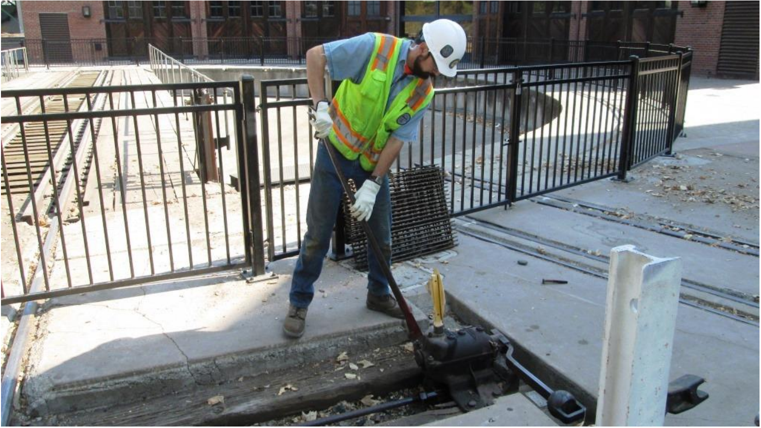
Matt pulls spikes on the switch machine at Switch 1
